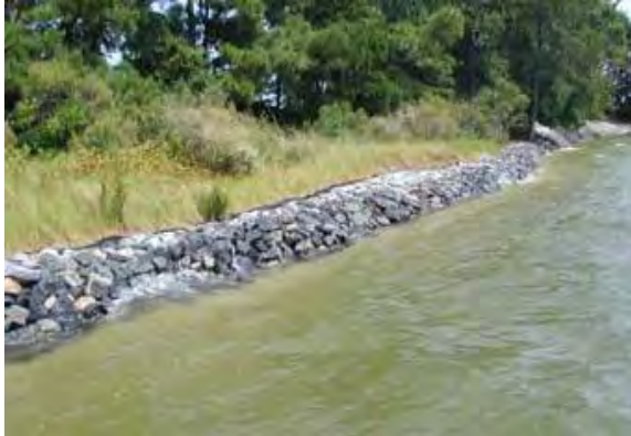
“marsh toe revetment”
